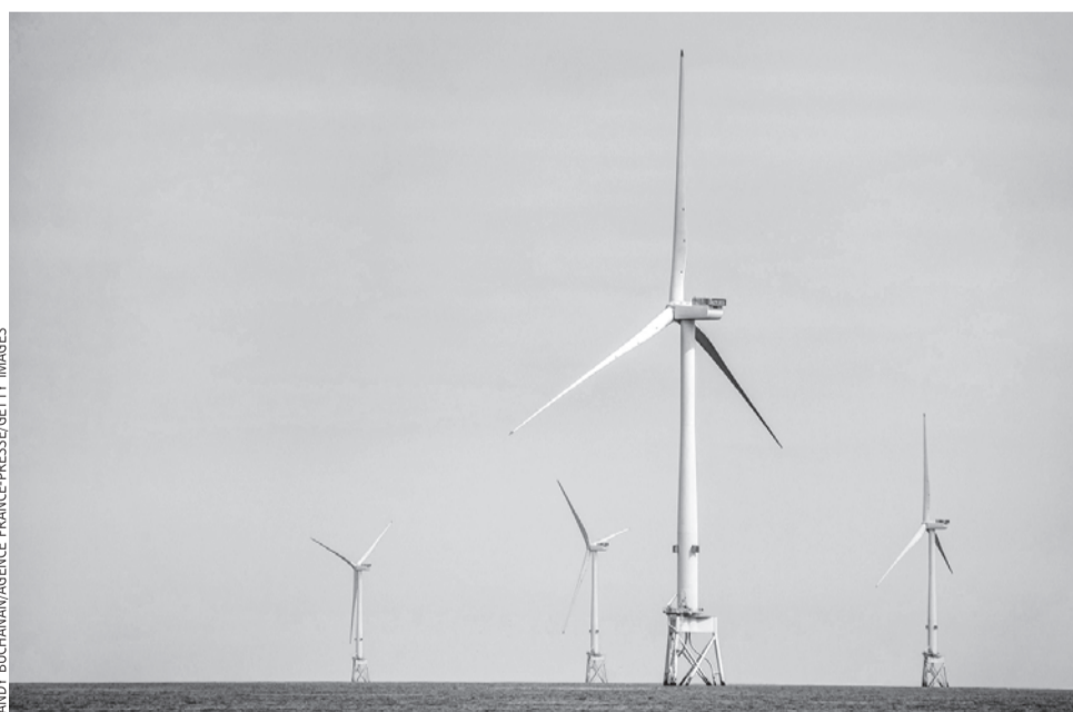
A wind farm under construction in the North Sea. Europe is seeing some wind-project delays.
