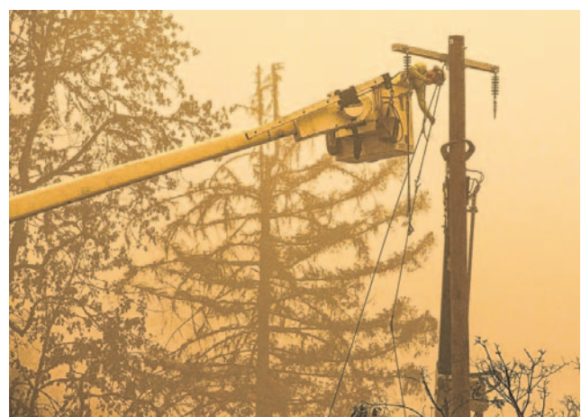
A utility worker did repairs amid wildfires in Oregon in 2020.
