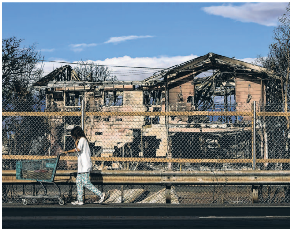
A home destroyed by the fire along the Honoapiilani Highway in Lahaina, Hawaii. At least 114 people died in the blaze in Lahaina, the deadliest U.S. wildfire in more than a century.
