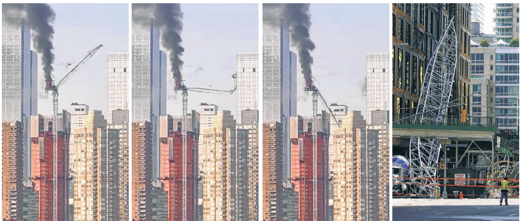
HIGH-RISE DRAMA: The engine compartment of a construction crane on the West Side of Manhattan caught fire Wednesday morning, the Associated Press reported, causing the arm of the crane, which was carrying a 16-ton concrete load, to snap off, smash against a nearby building and plunge to the street. Several people suffered minor injuries, officials said.
