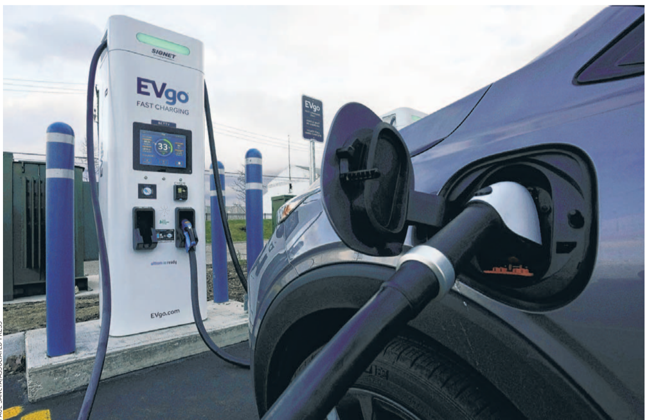
The U.S. will require an influx of fast chargers to support the expected surge in plug-in vehicles on the nation's roads.
