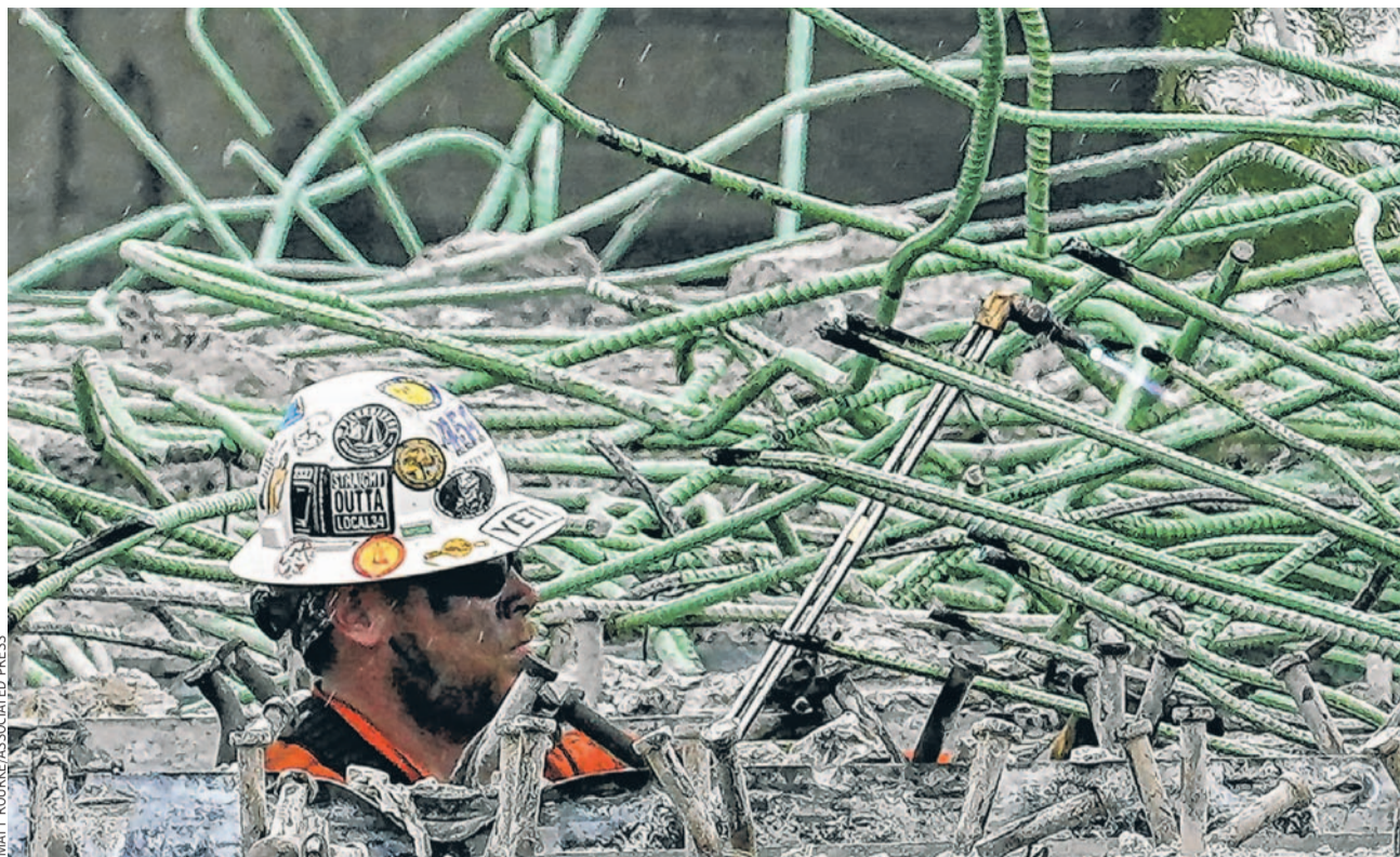
TRAFFIC SNARL: Pennsylvania officials said Wednesday that 2,000 tons of lightweight glass nuggets will be used to help rebuild and reopen a collapsed section of Interstate 95 in Philadelphia. Above, a worker cuts mangled reinforcing bars there.
