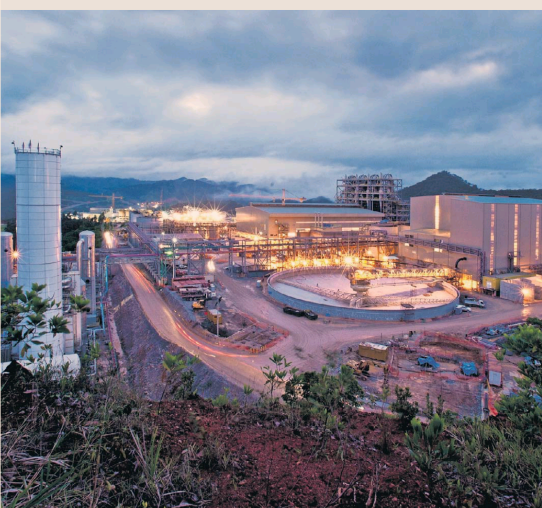
Plant commissioning at the Dominican Republic's Pueblo Viejo site helped push Barrick's earnings down
