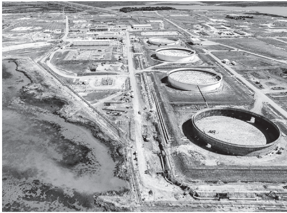
The U.S. is seeking to refill its Strategic Petroleum Reserve. A storage site in Freeport, Texas.
