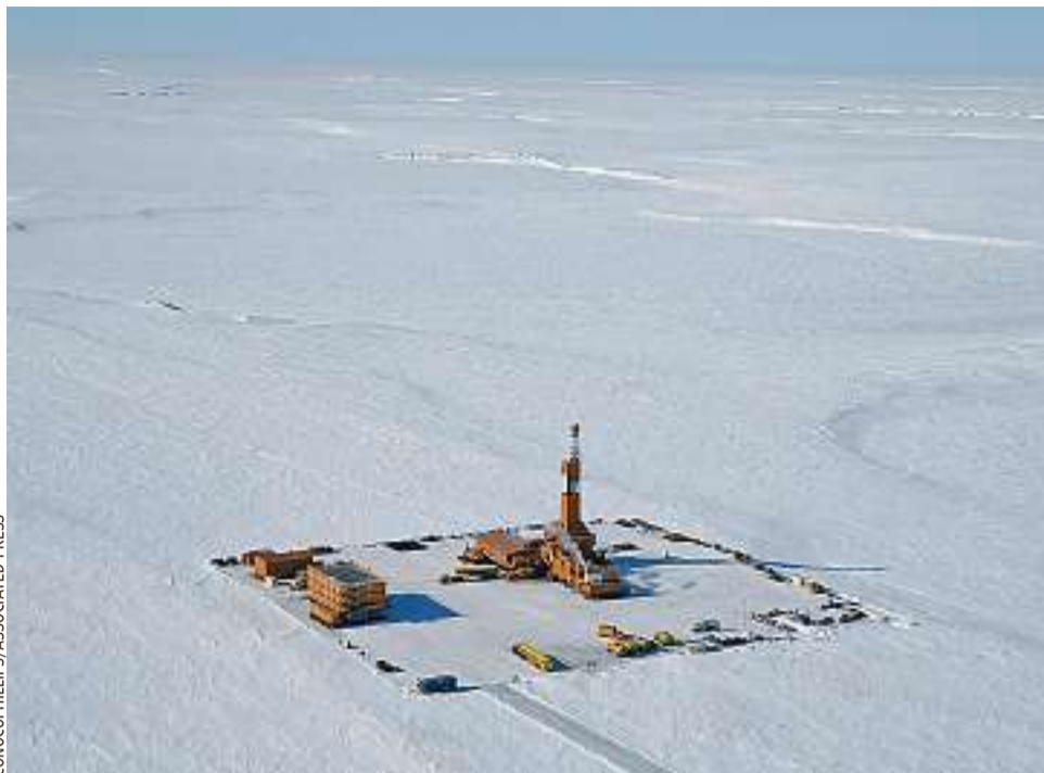
The site of the Willow oil project on Alaska's North Slope, which President Biden has greenlighted.
