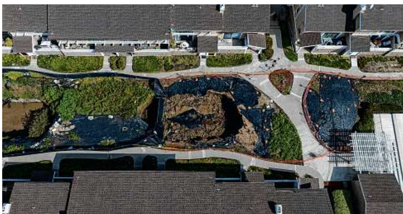
STORM EFFECTS: The atmospheric rivers plaguing California caused a 30-foot sinkhole near a condo complex in La Habra this week.
