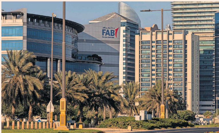
The scale of First Abu Dhabi Bank's international ambitions was only revealed alongside news it had been working for almost a year to buy StanChart and create a lender with more than $1tn in assets
