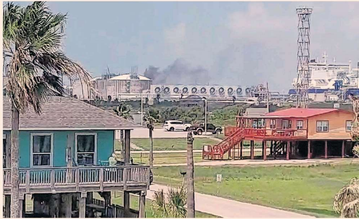
Smoke billows from the key Freeport LNG facility. The blast in June knocked out a centrepiece of the US gas export industry
