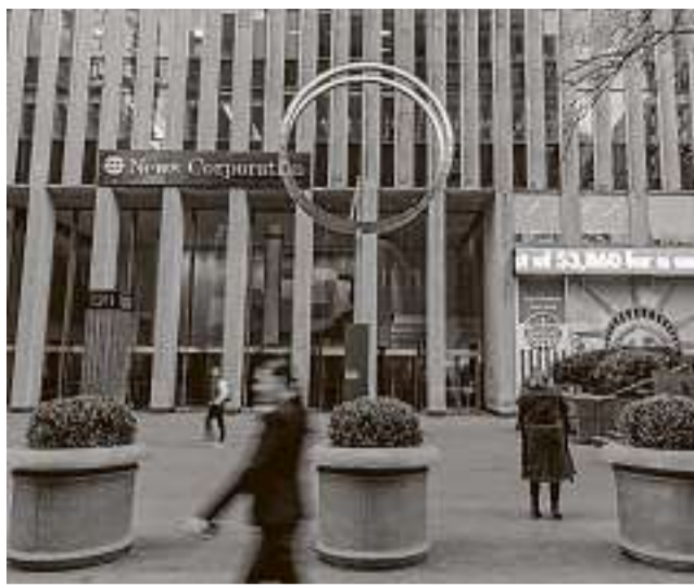
The leases include renovations to the lobby and outdoor plaza.
