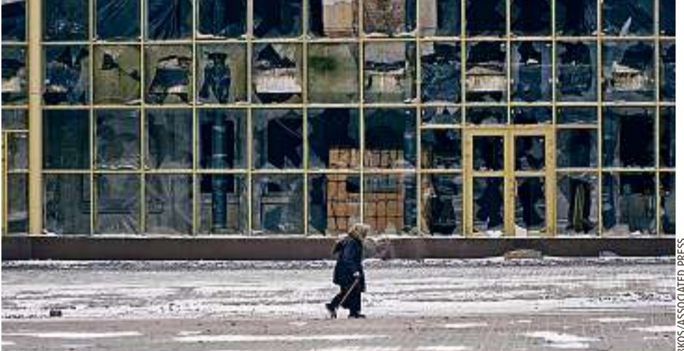
A local resident walks past damaged buildings in Bakhmut, Ukraine, on Thursday. In Moscow, a change in military leadership in the war efforts could signal a fresh Russian offensive. A16
