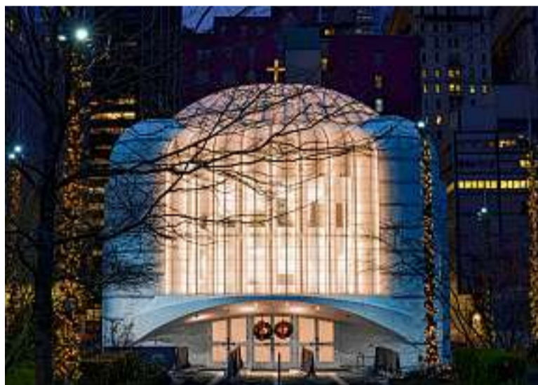
The exterior of the structure illuminated at night
