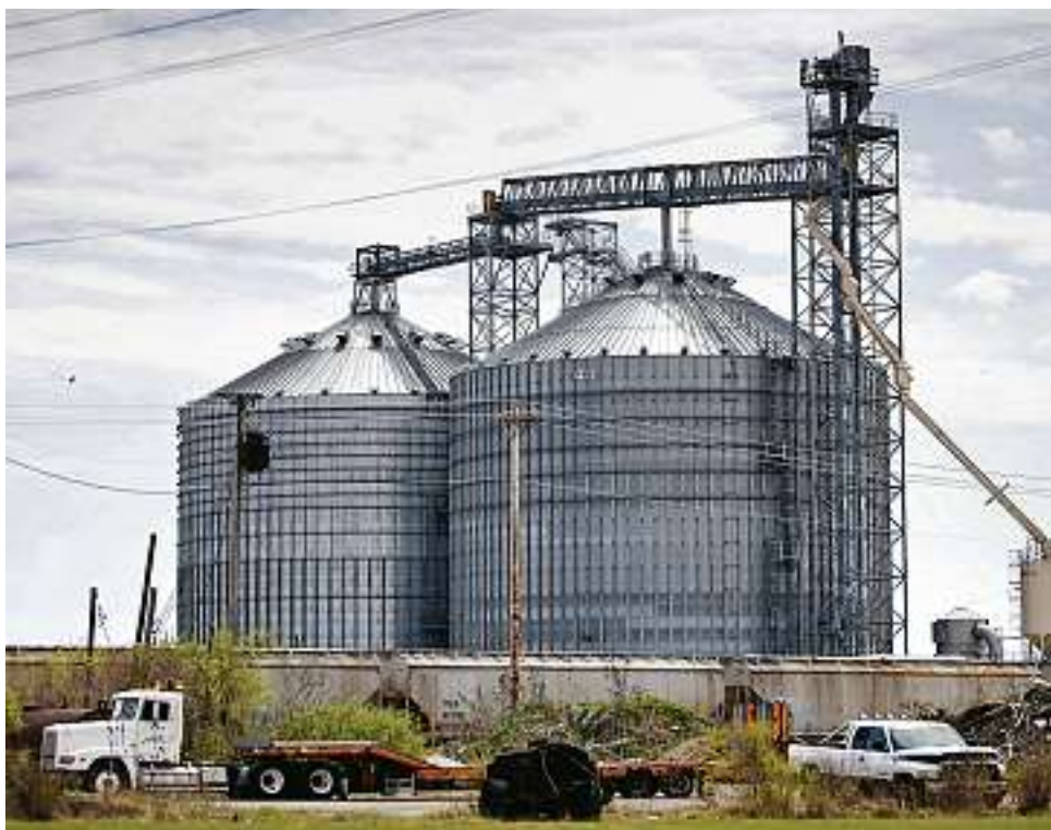
The company buys crops, trades commodities and processes meat. A Cargill soybean facility.
