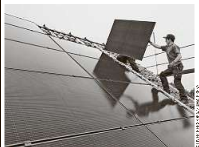
A workman installs solar panels on the roof of a residence.
