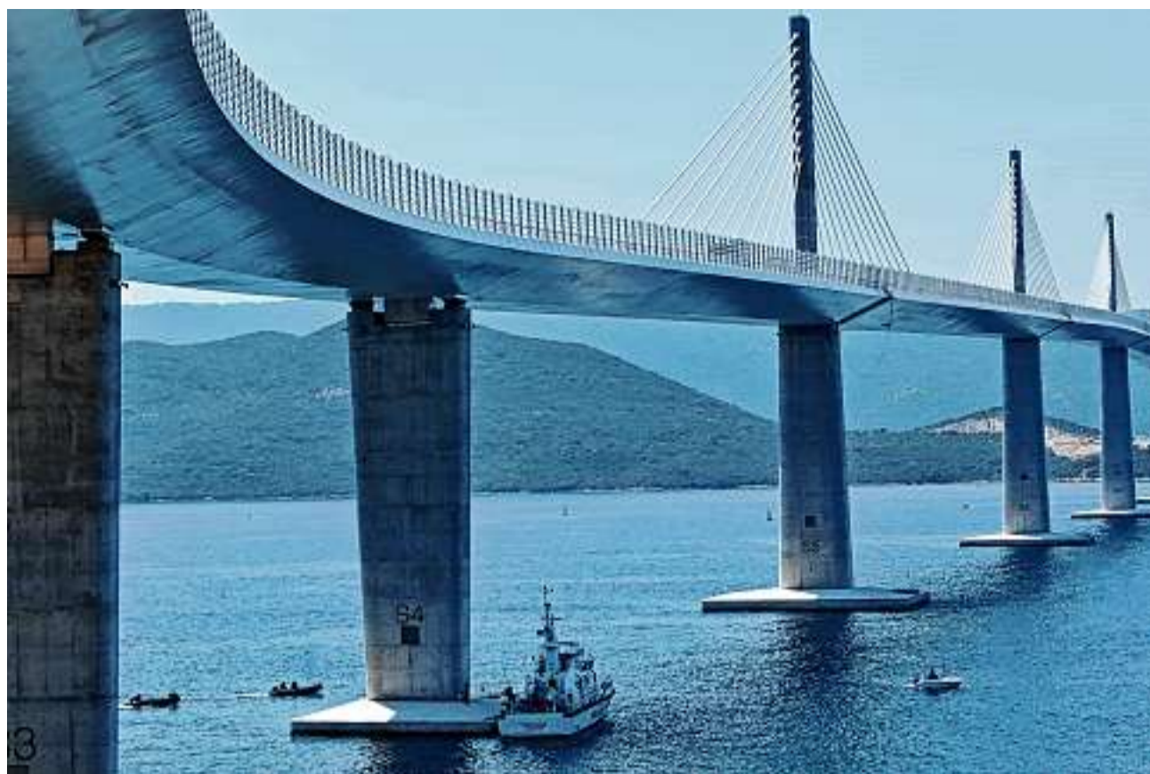
State-owned China Road & Bridge built the Pelješac Bridge in Croatia after its 2017 bid came in at a discount to rival proposals.
