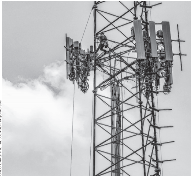
Crown Castle owns wireless towers and fiber-optic lines.
