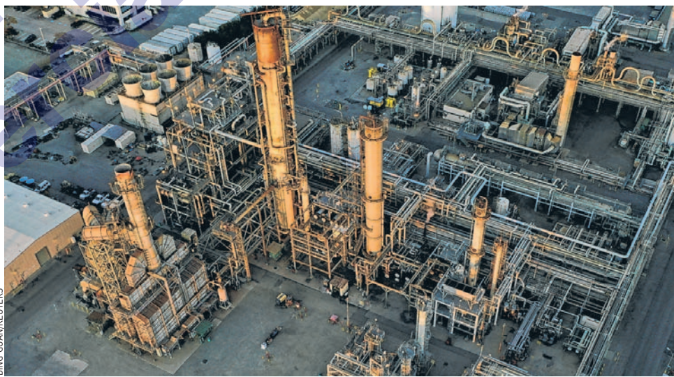
The oil refiner named former Cenovus executive Robert W. Pease to its board.
