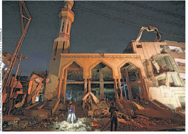
A destroyed mosque in Rafah after air strikes early Monday.
