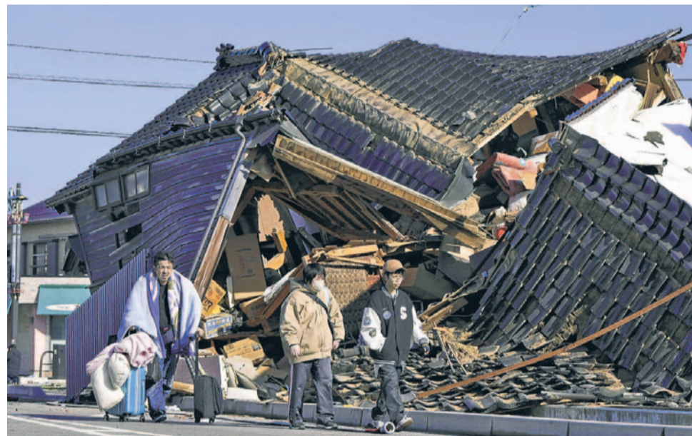
A deadly magnitude-7.6 quake destroyed homes and buildings in Wajima, Ishikawa prefecture,
