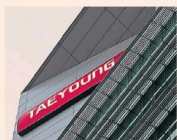
Analysts caution that Taeyoung's liquidity crunch could spread
