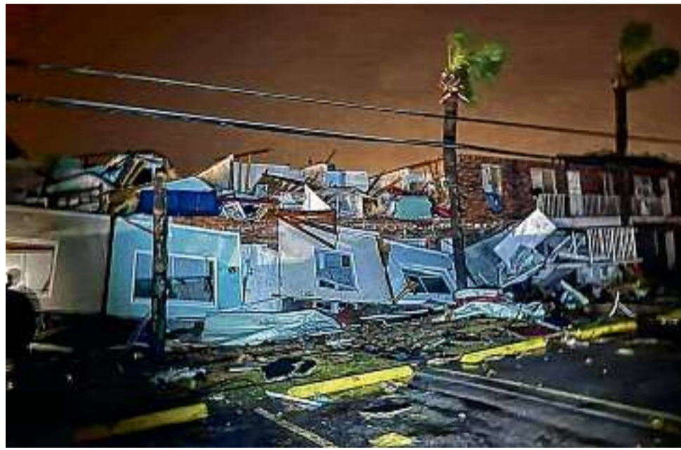
Storm damage was visible around Panama City Beach, Fla., early Tuesday.
