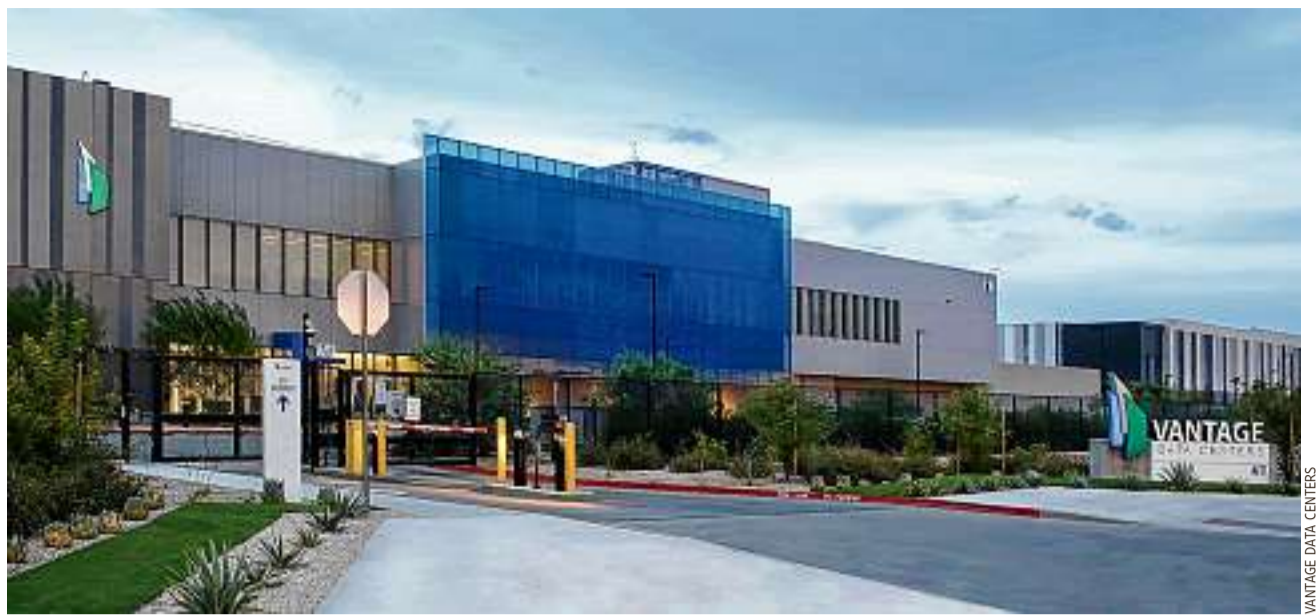
Vantage Data Centers has 32 campuses around the world to meet growing demand from tech companies. A facility in Arizona.
