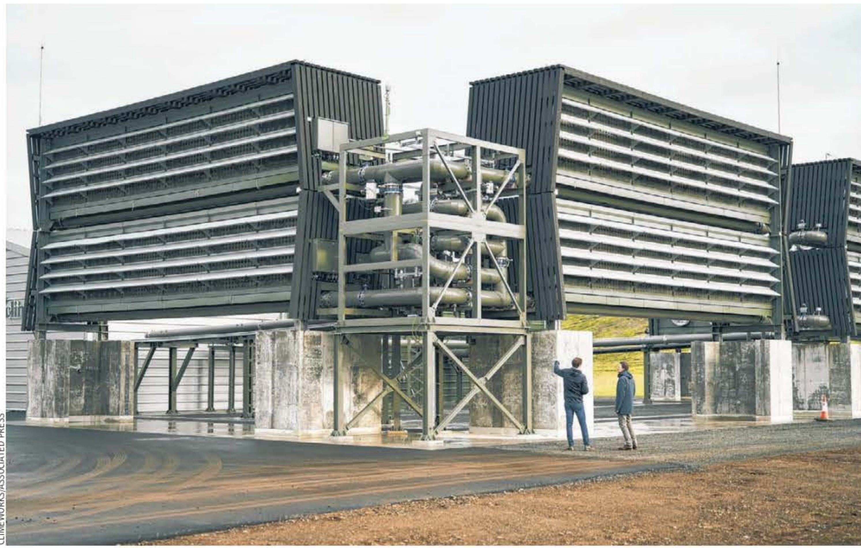
A Climeworks plant near Reykjavik, Iceland, where an air-scrubbing machine sucks air into boxes that filter out carbon dioxide.
