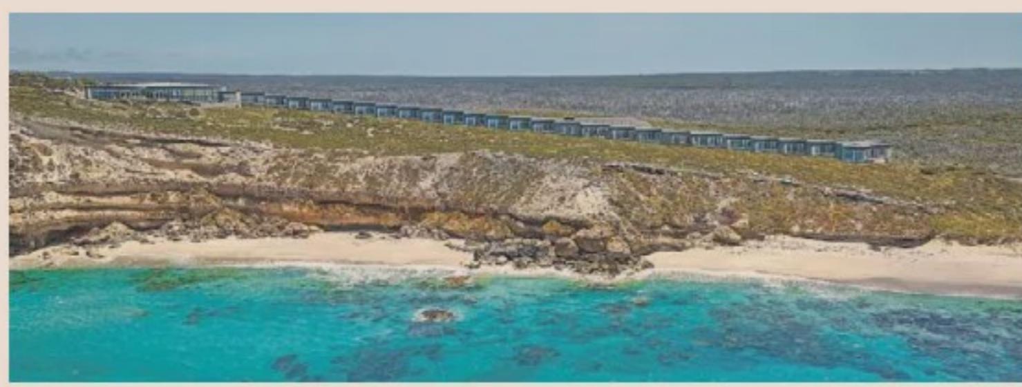
Below: the suites form a subtly bending line that descends towards the beach George Apostolidis
