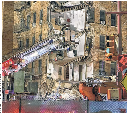
Firefighters searched the rubble where a six-story corner of a Bronx apartment building collapsed on Monday.
