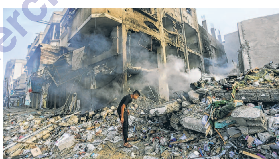
Buildings in Khan Younis in the southern Gaza Strip were destroyed during Israeli airstrikes.
