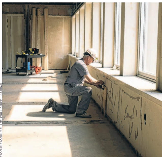
An office-to-apartment conversion project in Minneapolis.
